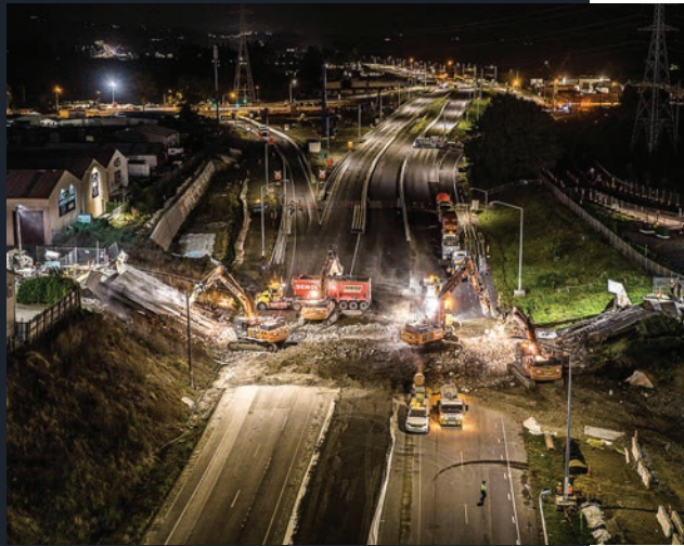
SH1 Papakura to Drury upgrades under construction.
